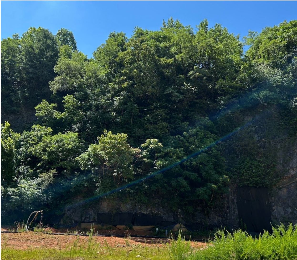
Figure 11. Vegetation Growth on Quarry Sidewalls
