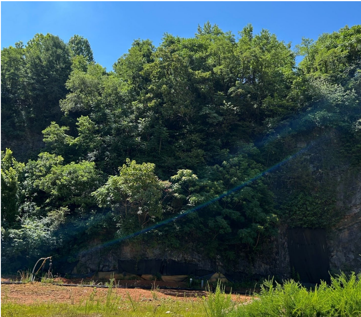
Figure 11. Vegetation Growth on Quarry Sidewalls
