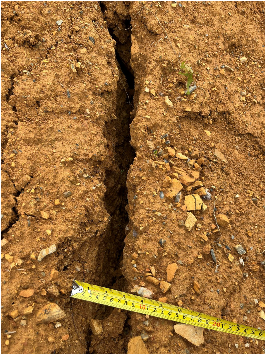
Figure 3. Settlement Crack Observed in Southwest Area Near Sidewall Bench
