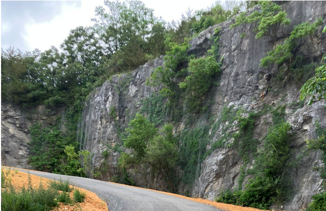
Figure 12. Vegetation Growth on Quarry Sidewalls
