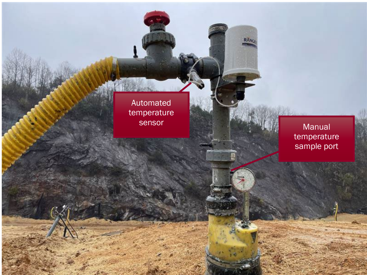
Figure 2. Typical LFG Extraction Wellhead with Automated Temperature Probe
