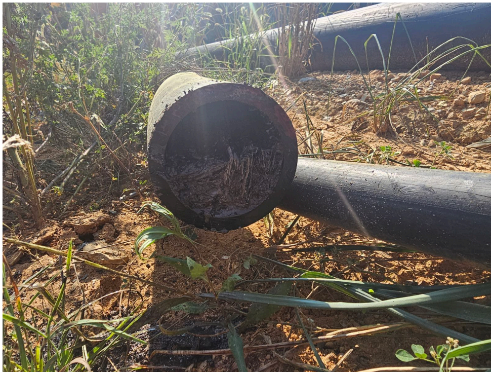
Figure 15. Solids in Landfill Gas Liquids Forcemain
