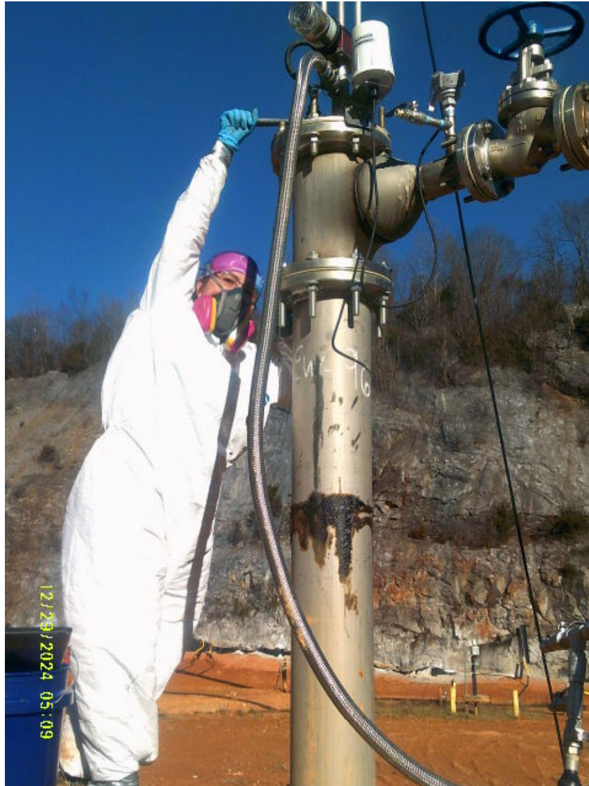
Figure 15. Technician Attempting to Access EW-96
