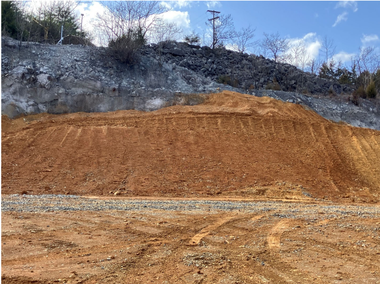
Figure 4. Soil Placed Against the Sidewall
