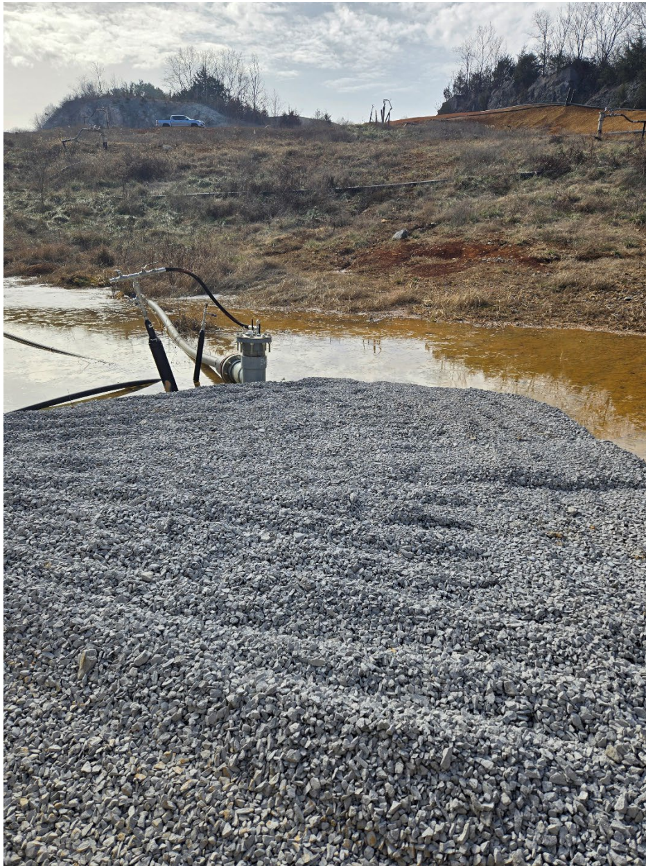
Figure 15. Conditions at EW-70 after Aggregate Installation
