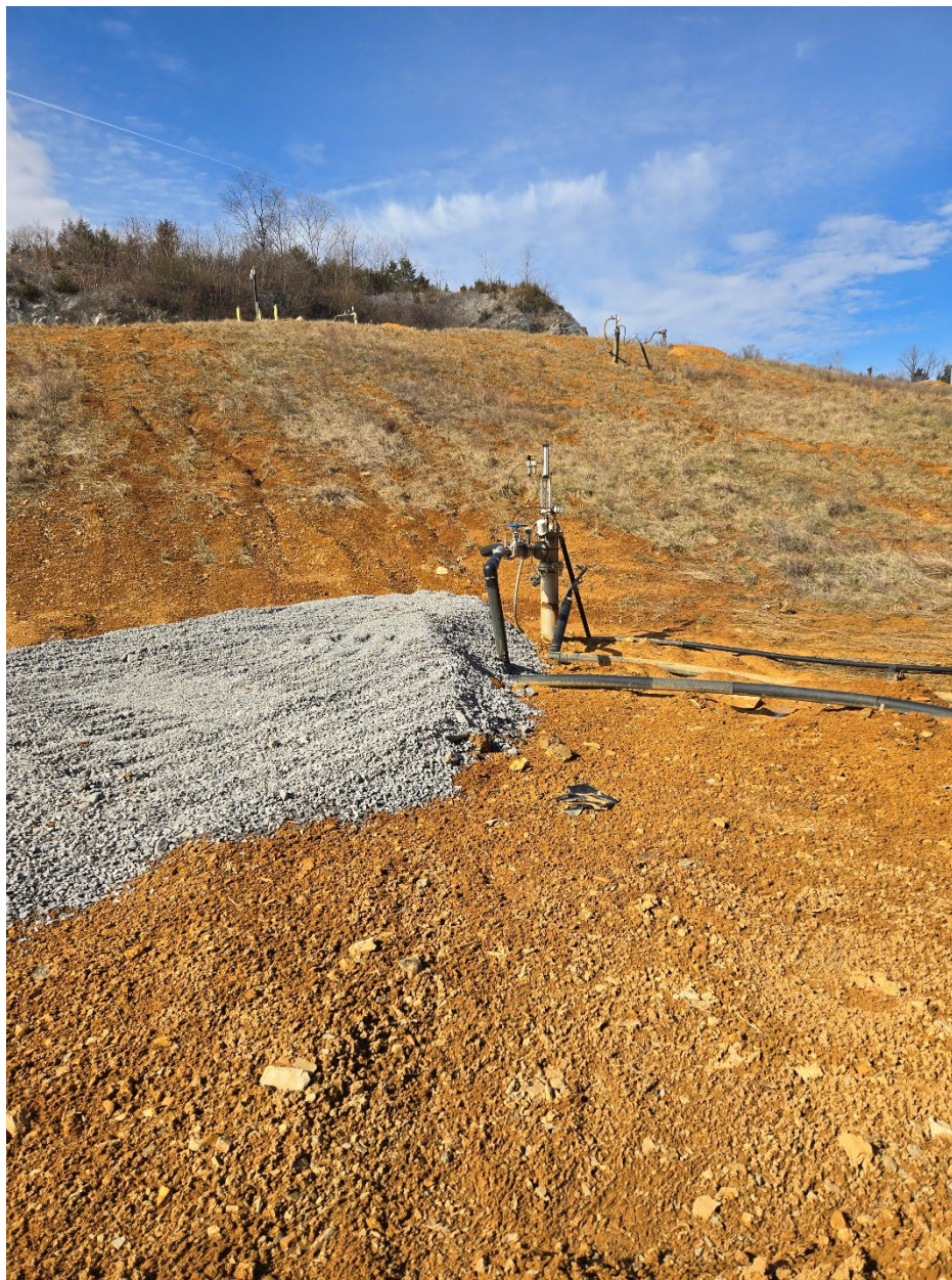
Figure 17. Conditions at EW-82 after Aggregate Installation
