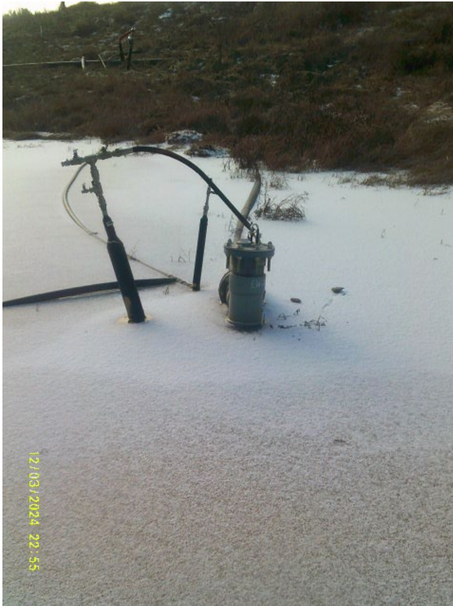
Figure 14. Conditions at EW-70 During Liquids Sampling Event
