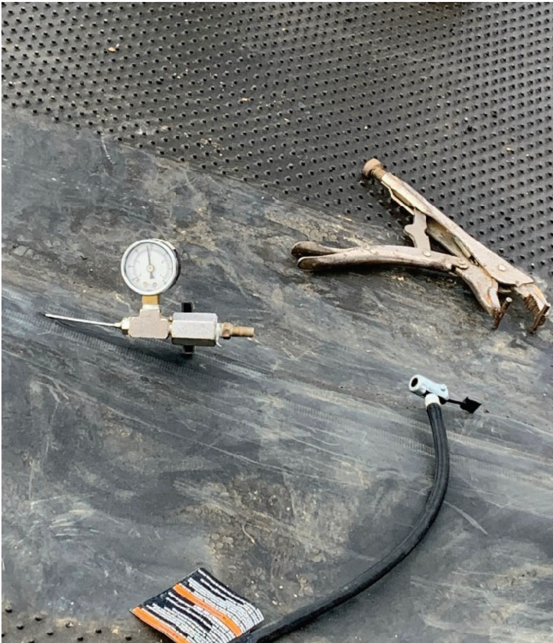
Figure 6. Air Pressure Testing of Geomembrane Seam
