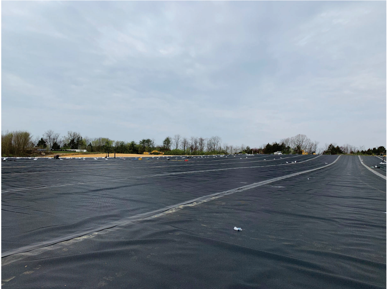
Figure 5. Geomembrane Installation on March 22 nd
