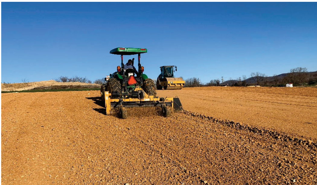
Figure 4. Mechanical Raking of the Intermediate Cover Soil Surface
