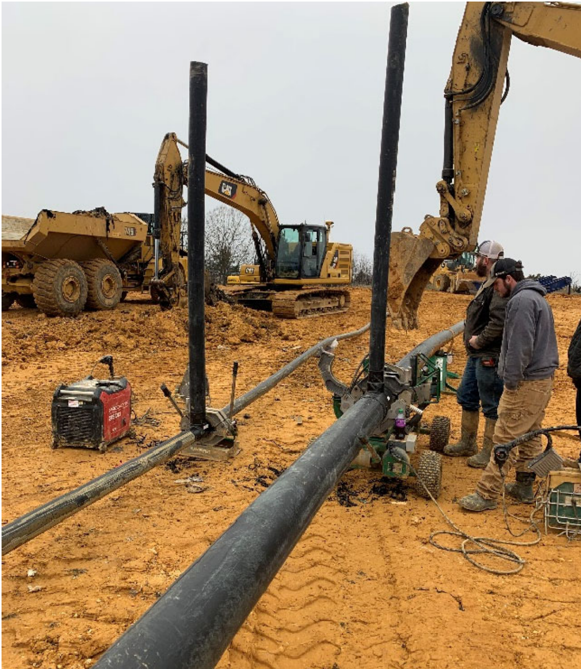
Figure 2. Landfill Gas Installation Progress - SWP No. 498 Landfill
