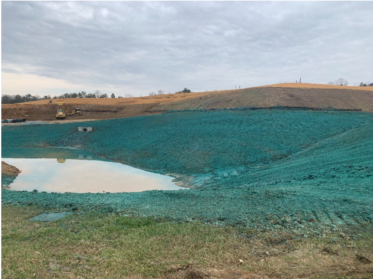
Figure 7. Stabilizing Stormwater Basin Area
