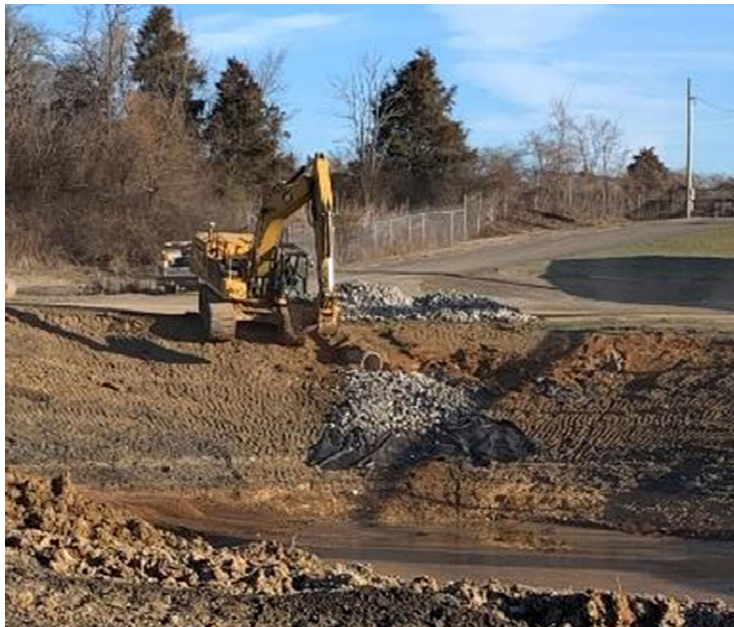
Figure 6. Installation of Outlet Protection in the Stormwater Basin
