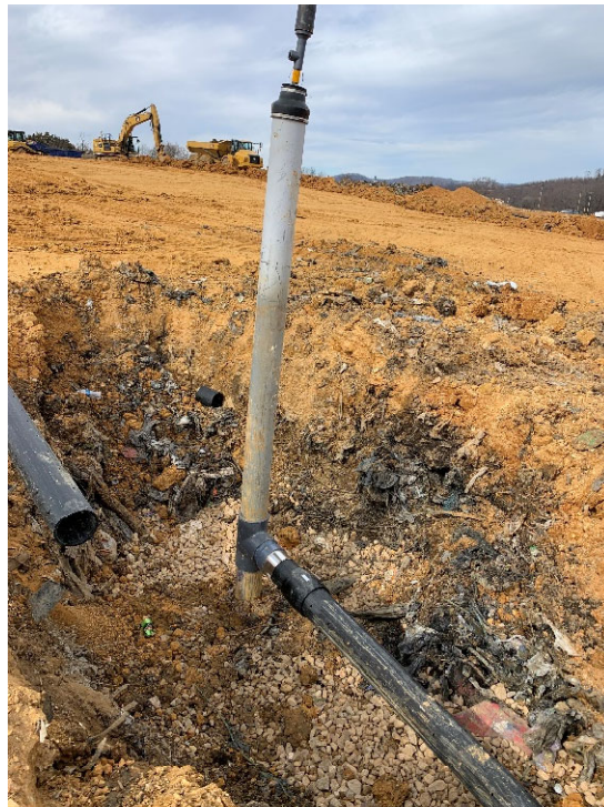
Figure 4. Horizontal Collector Wellhead and Drainage Pit Installation
