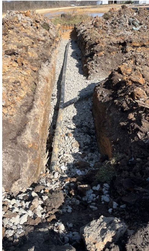
Figure 1. Construction of a Horizontal Collector and EW-16
