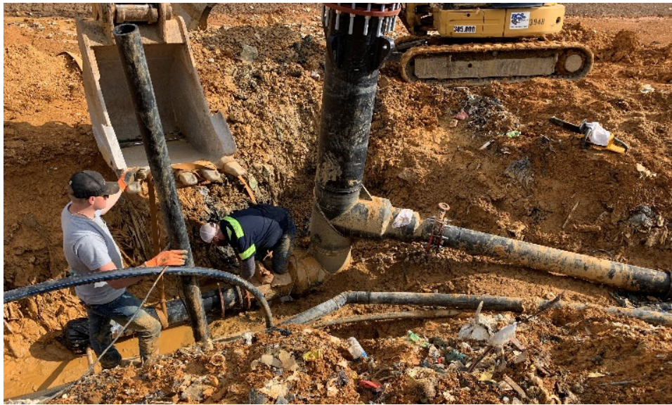
Figure 3. Landfill Gas Installation Progress - SWP No. 498 Landfill
