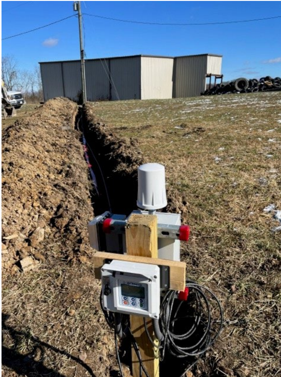
Figure 25. Flow Meter Installation
