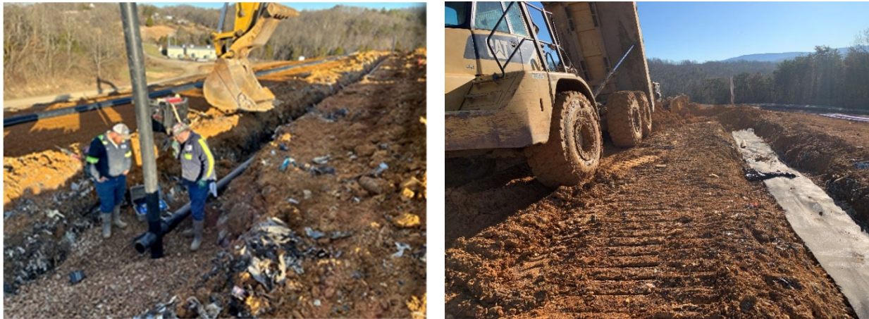
Figure 1. Landfill Gas Installation Progress - SWP No. 498 Landfill
