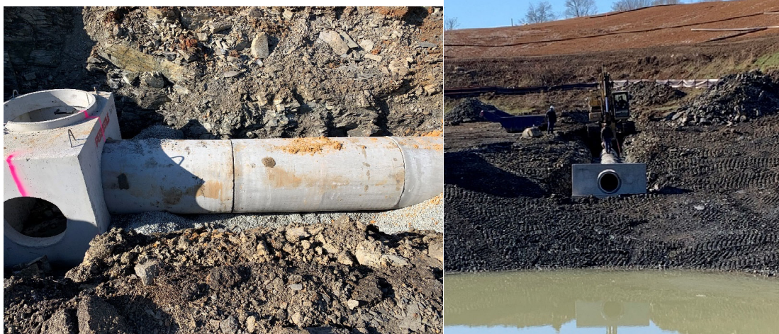
Figure 2. Installation of the Stormwater Sewer System - SWP No. 498 Landfill
