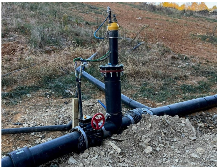
Figure 6. Sump CS-3 Installation at the SWP No. 588 Landfill
