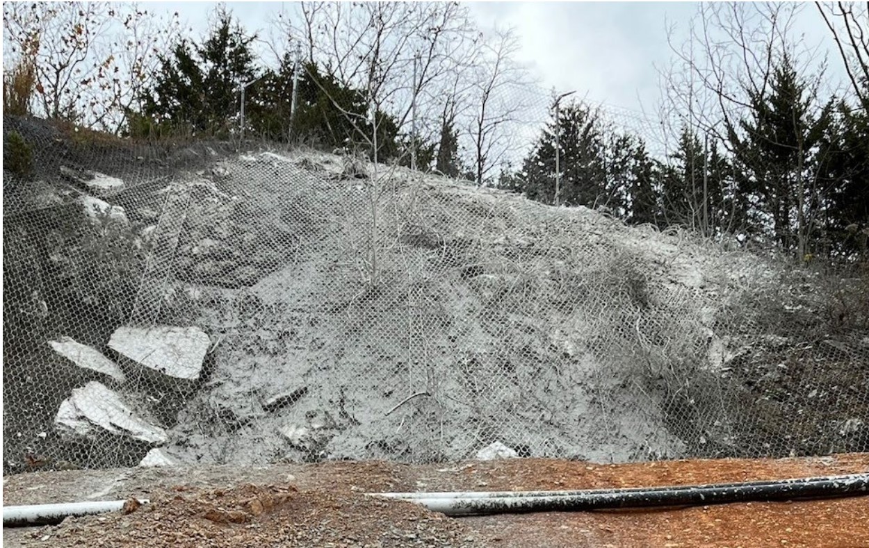
Figure 11. Phase 2 SOMS Lower and Upper Collector Construction Maintenance
