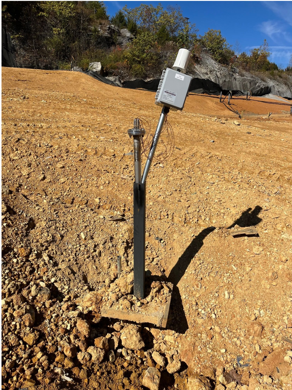
Figure 18. Damage to TP-5
