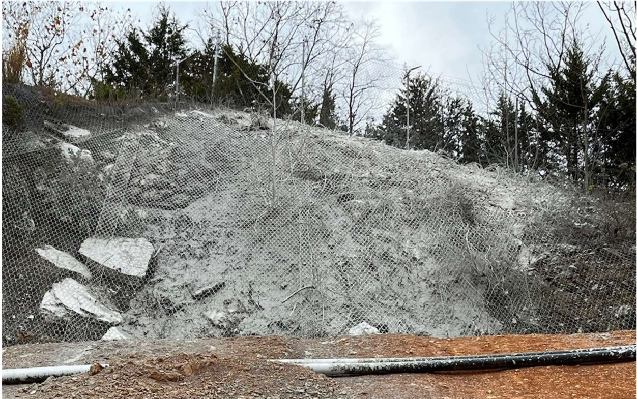
Figure 12. Phase 2 SOMS Lower and Upper Collector Construction Maintenance
