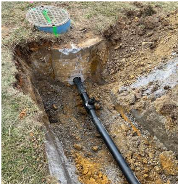
Figure 2. 4" HDPE connection to manhole at the SWP No. 588 Landfill
