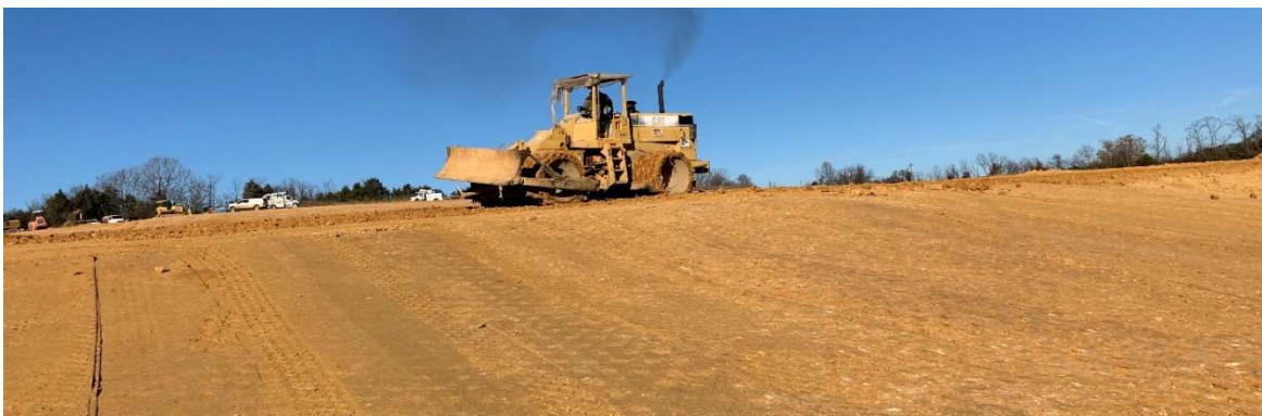
Figure 1. Grading Progress on the SWP No. 498 Landfill
