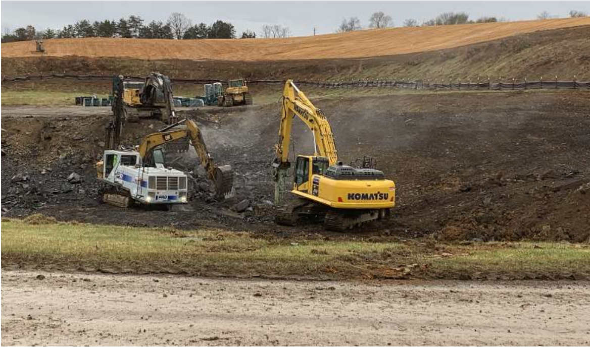
Figure 2. Excavation of the stormwater basin adjacent to SWP No. 498 Landfill
