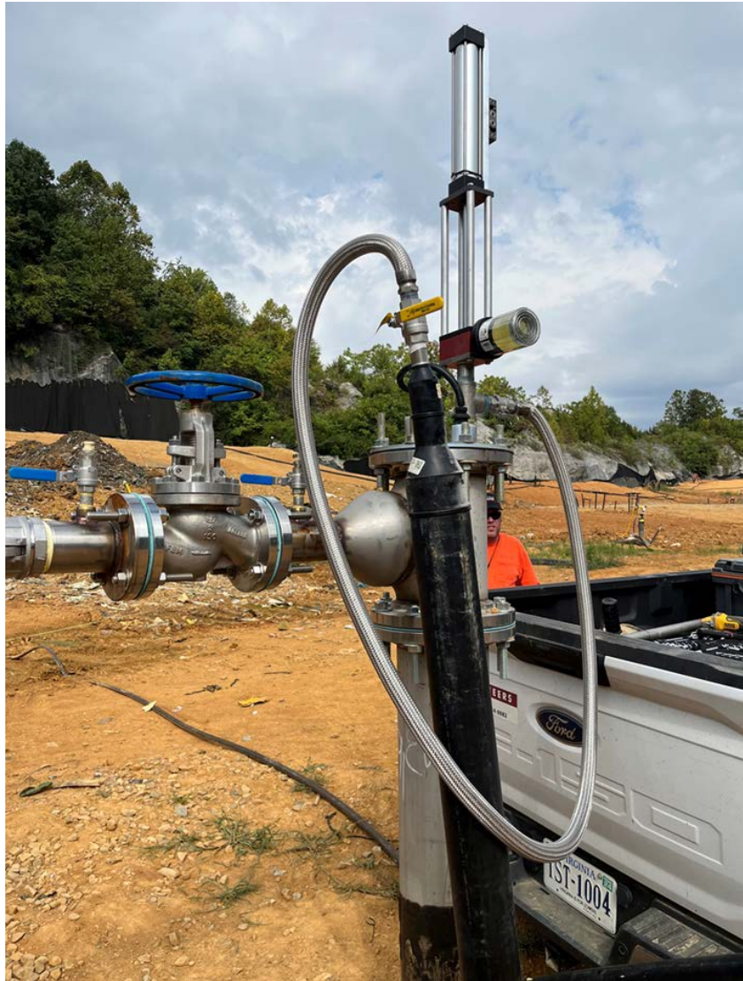
Figure 7. Extraction Well Pump Installation at the SWP No. 588 Landfill
