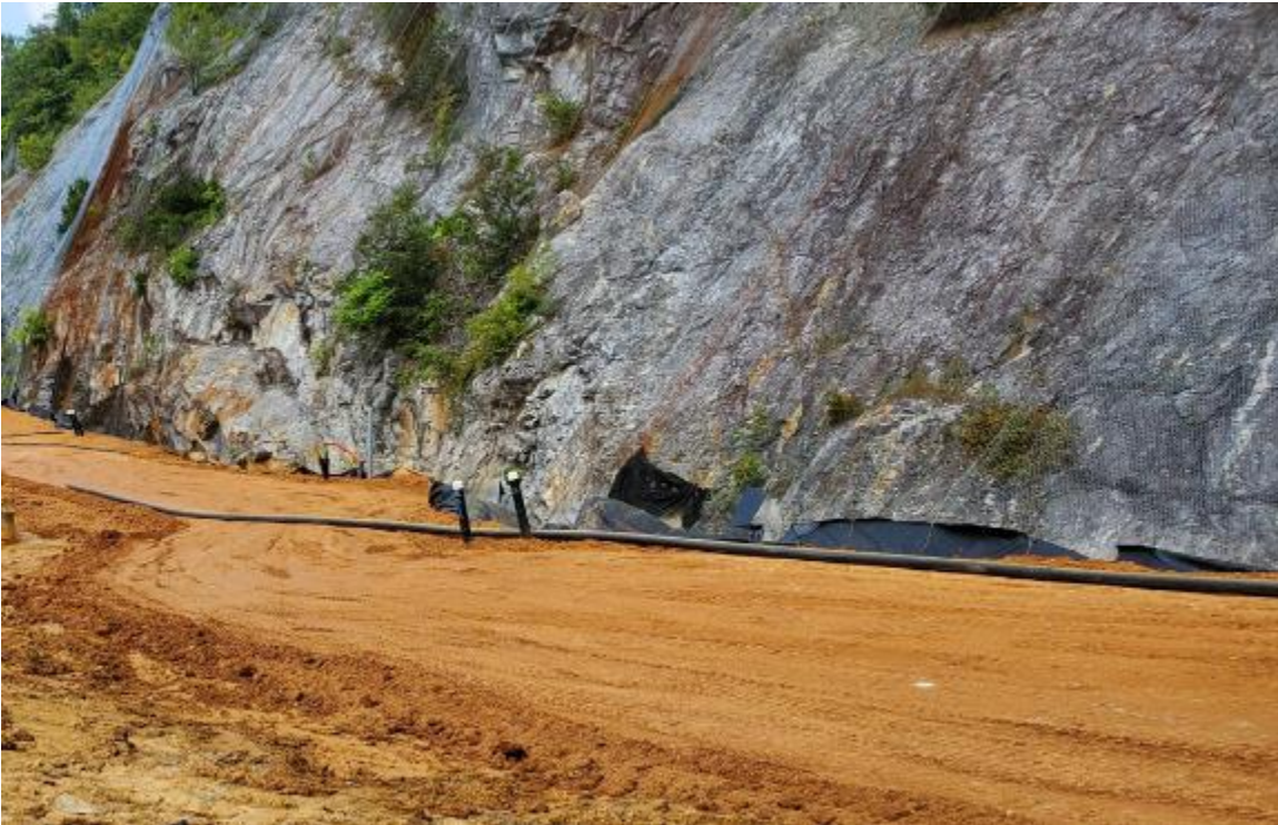
Figure 11. Phase 2 SOMS Lower and Upper Collector Construction
