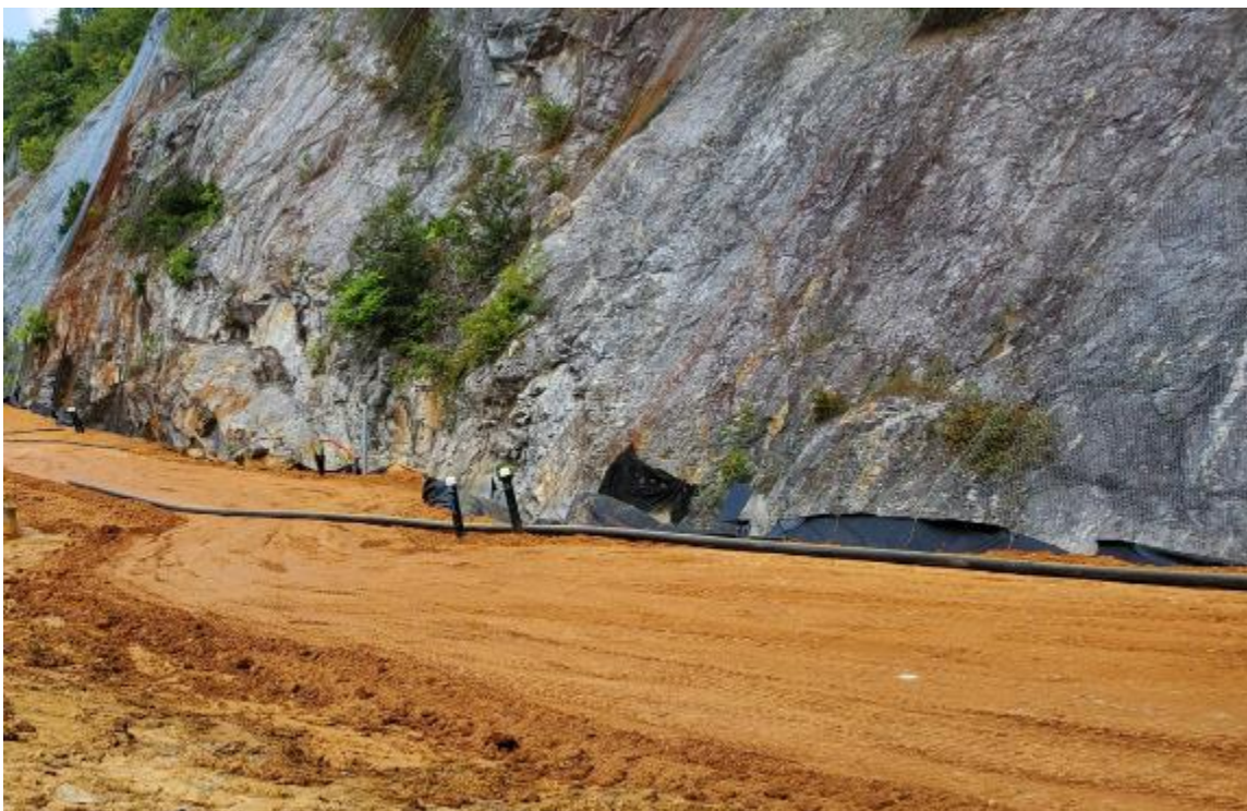
Figure 7. Phase 2 SOMS Lower and Upper Collector Construction
