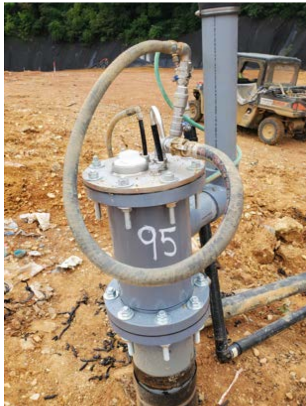
Figure 2. Extraction Well 95 Pump Installation at the SWP No. 588 Landfill
