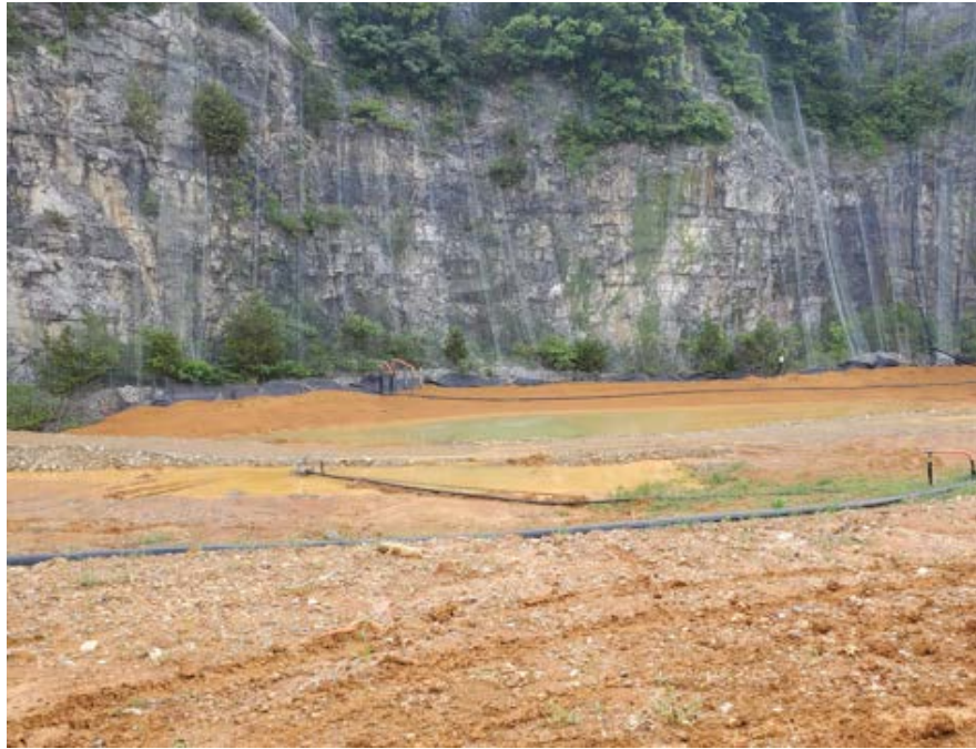
Figure 3. Stormwater Accumulation at the SWP No. 588 Landfill
