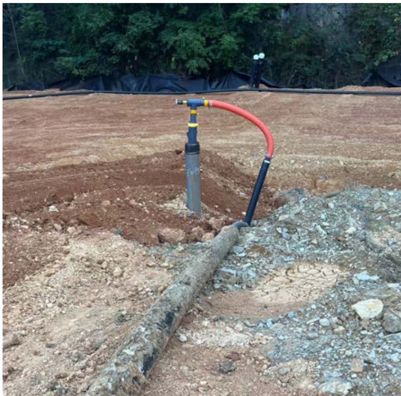
Figure 3. Extraction Well 85 Installation at the SWP No. 588 Landfill
