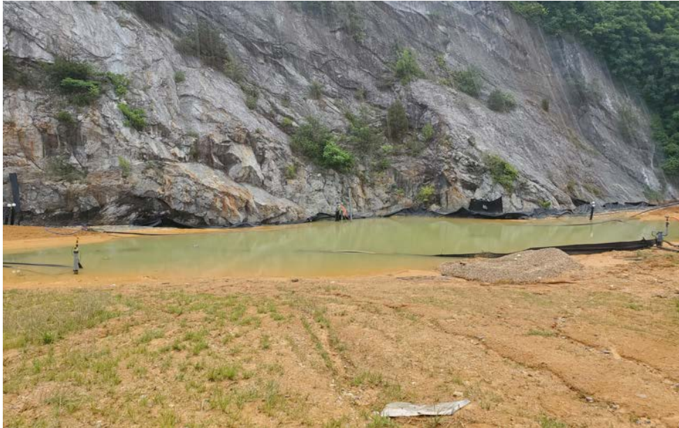
Figure 4. Stormwater Accumulation at the SWP No. 588 Landfill
