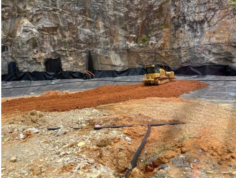
Figure 8. Phase 2 SOMS Lower and Upper Collector Construction
