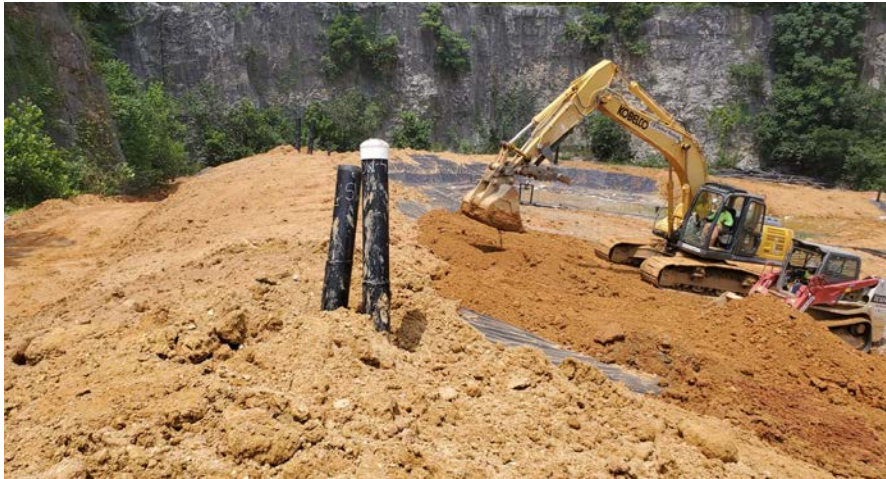
Figure 5. Phase 2 SOMS Lower and Upper Collector Construction
