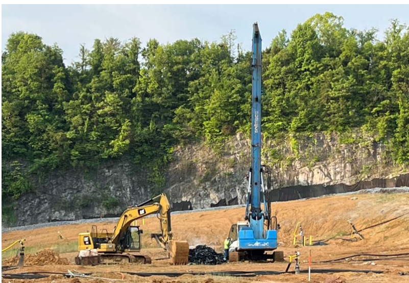
Figure 1. Deep-Well Drilling at the SWP No. 588 Landfill
