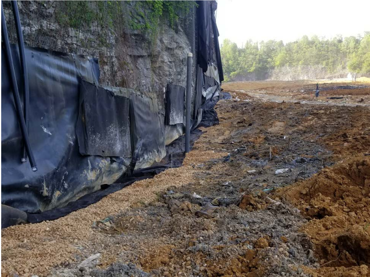
Figure 6. Phase 2 SOMS Lower Collector Construction
