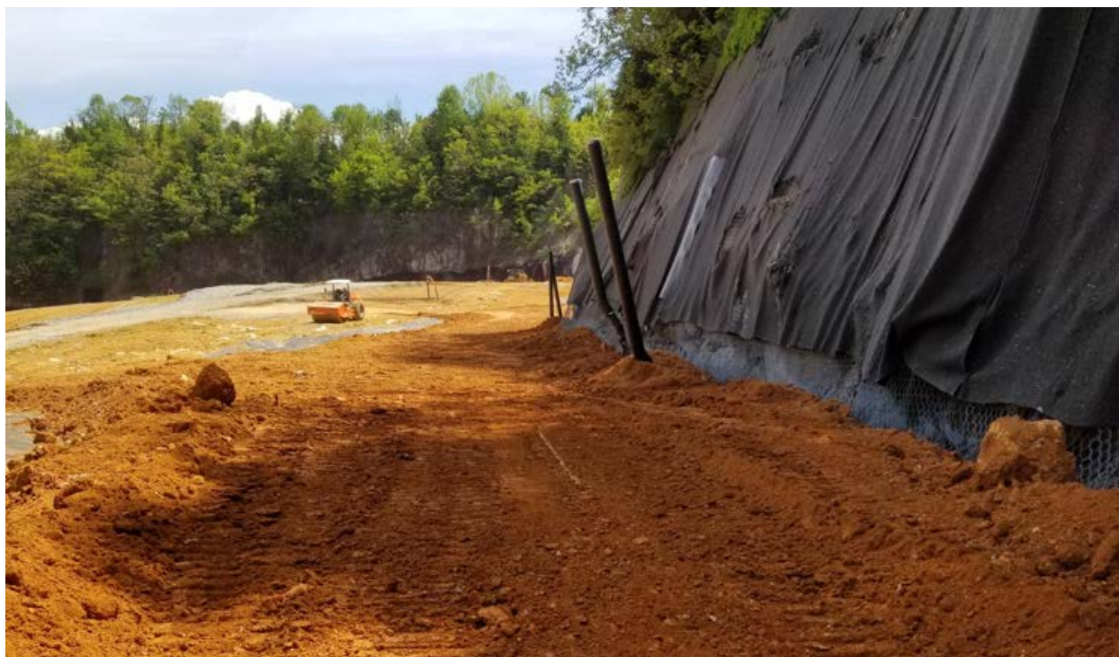
Figure 4. Phase 2 SOMS Low Permeability Soil Placement
