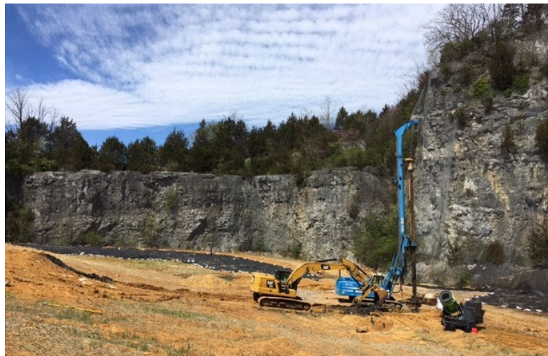
Drilling EW-70, installed SOMS liner in the background
