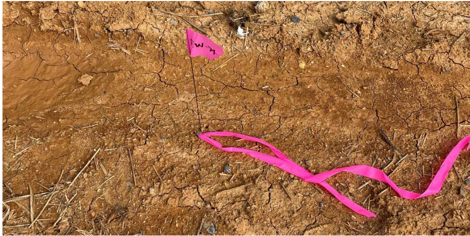
Figure 1. Proposed Landfill Gas Collect Well Location Marker
