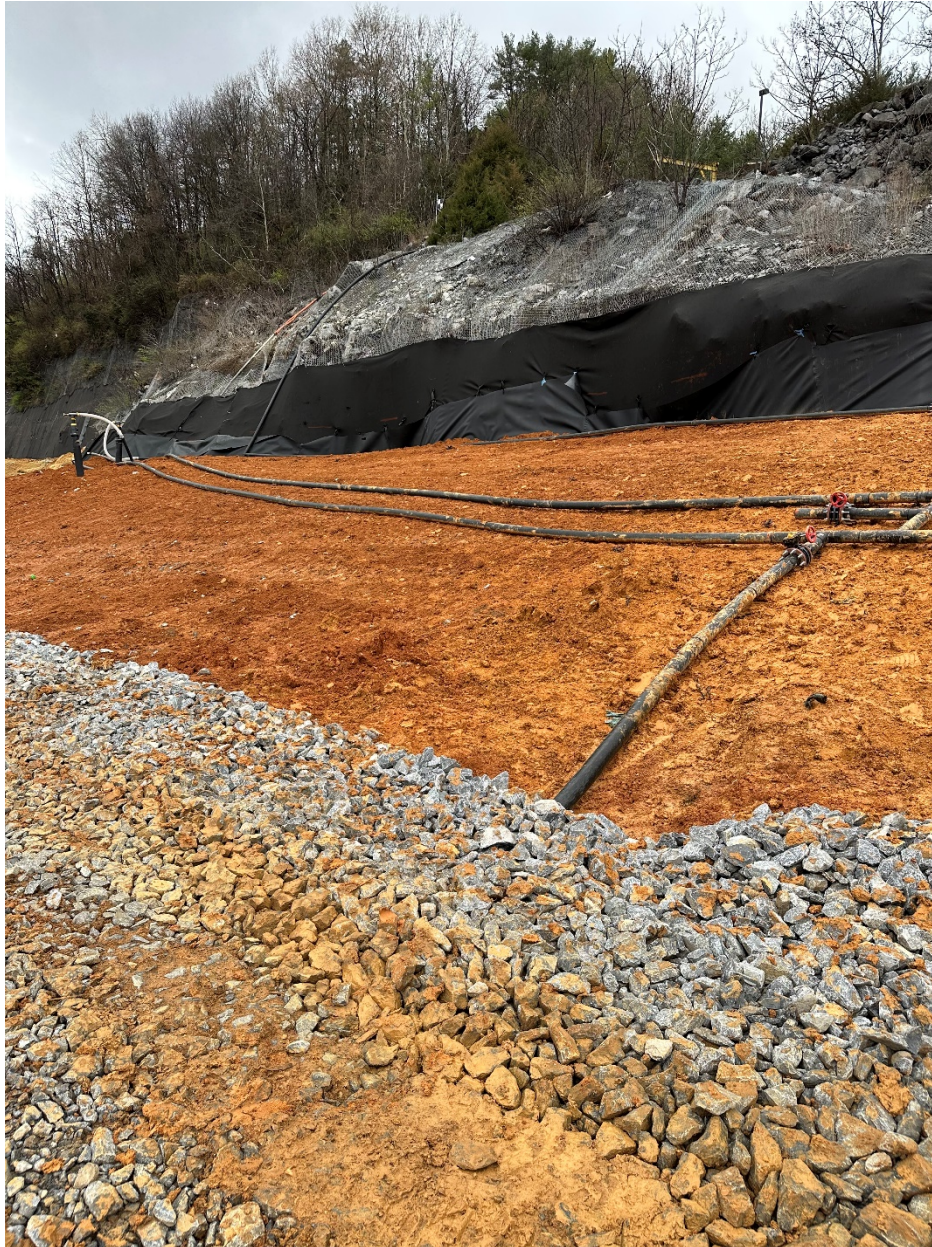
Figure 8. Phase 1 Sidewall Odor Mitigation System Construction
