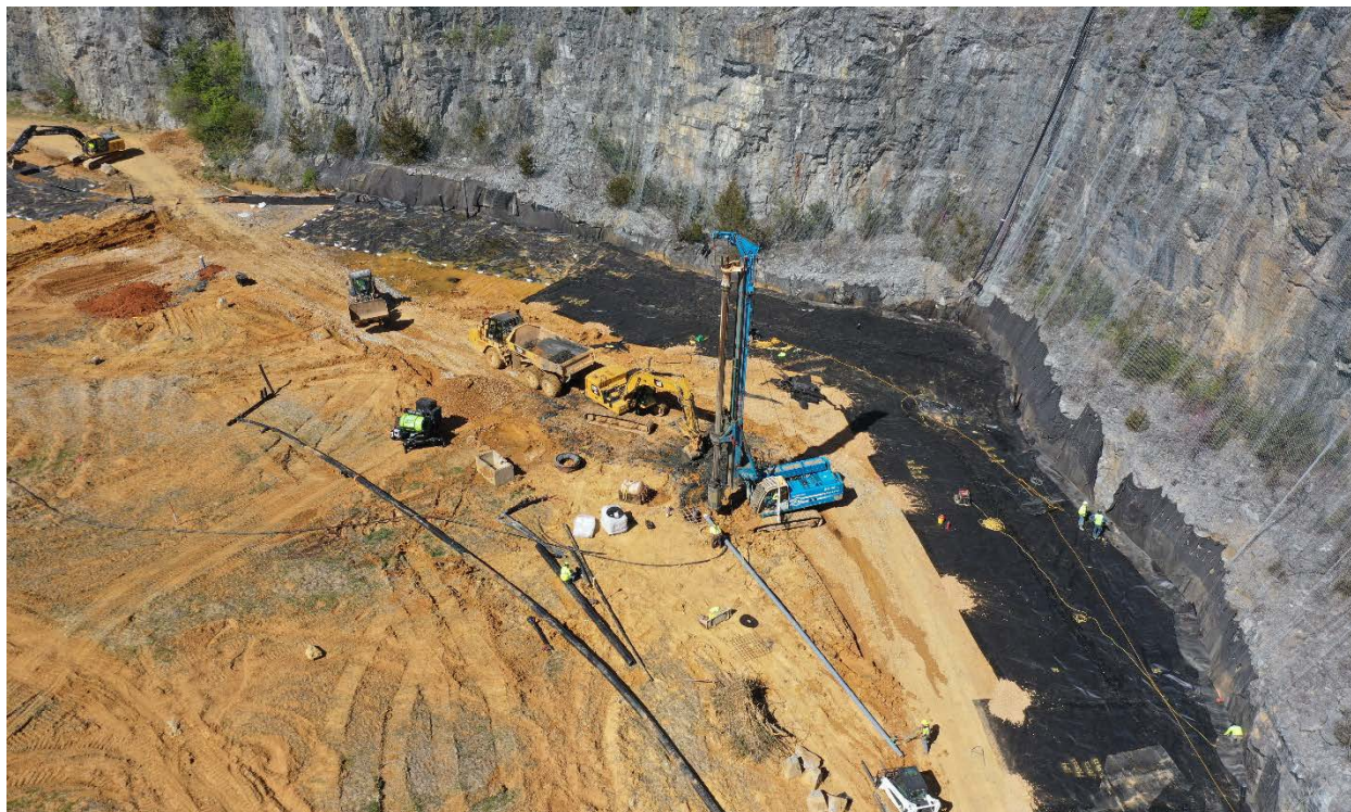
Figure 5. Landfill Gas Extraction Well Drilling
