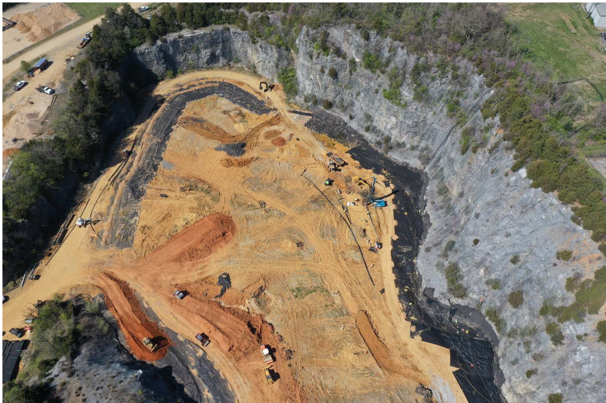
Figure 9. Phase 2 SOMS Construction
