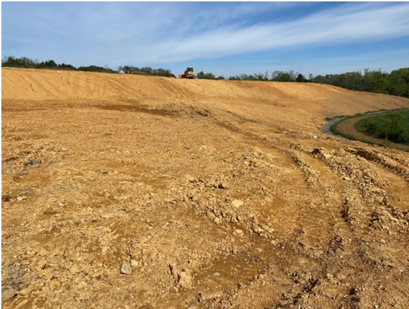
View of landfill surface showing slope and grade for positive drainage.
