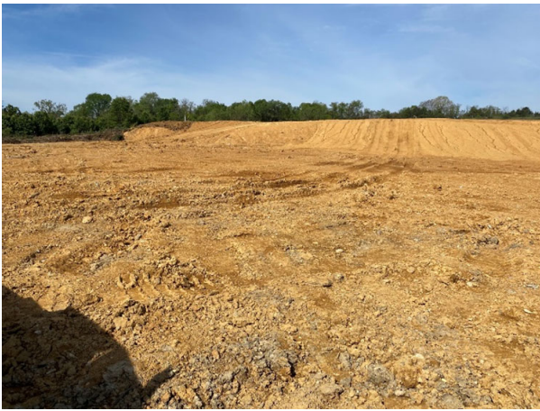
View of top of landfill showing positive drainage looking west.
