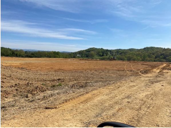
View of top of landfill surface.
