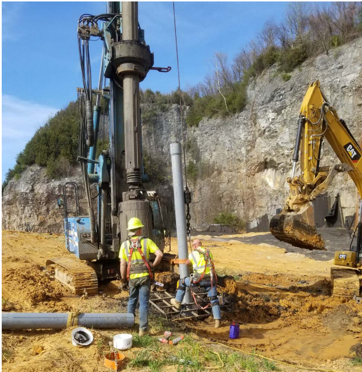
Figure 2. Landfill Gas Extraction Well Drilling Operations
