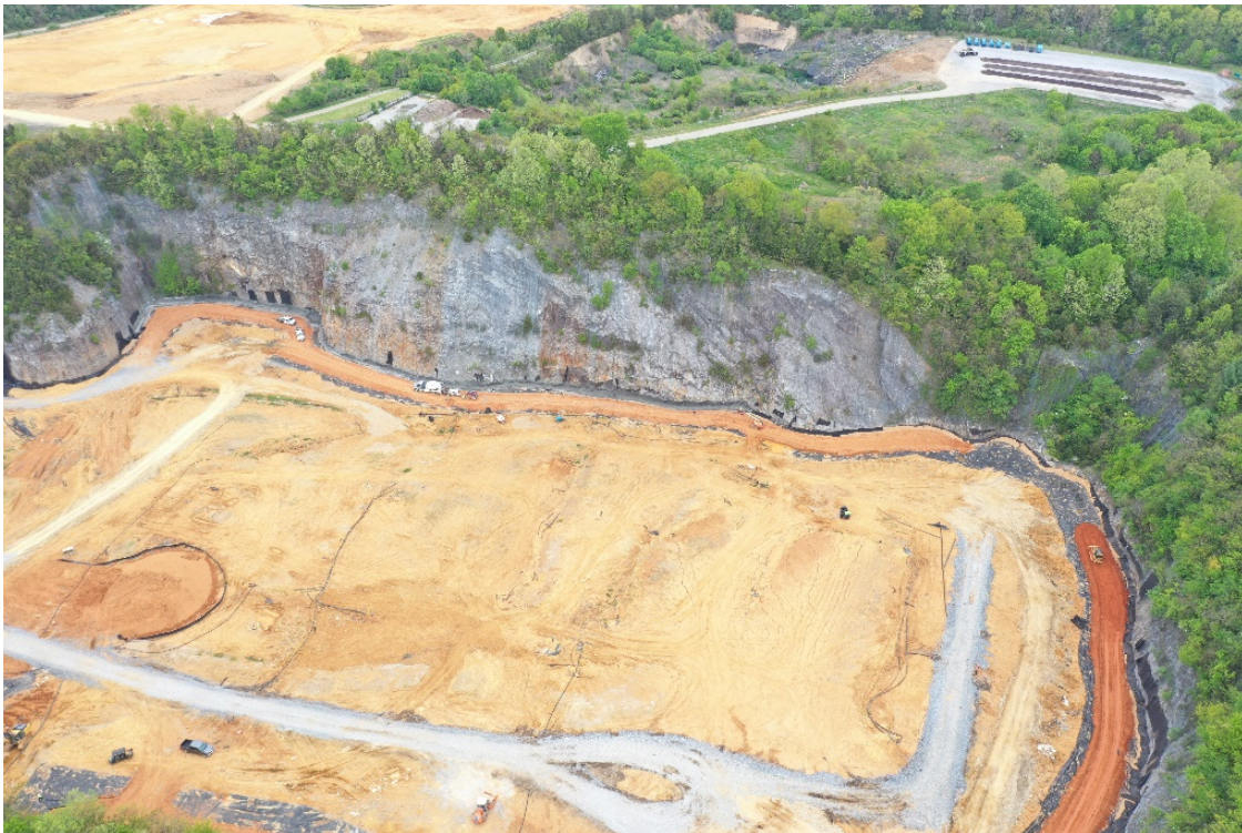
Figure 5. Phase 2 SOMS Construction
