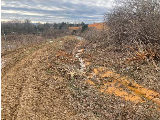
Stormwater diversion channel and trench berm prior to clean-out and stabilization.
