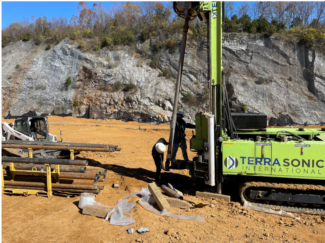
Figure 5. Temperature Monitoring System Drilling
