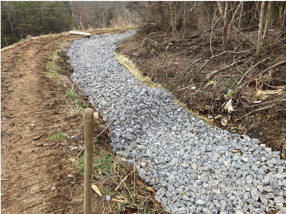
Figure 2. Stormwater Diversion Channel/Trench Berm Work Progress
