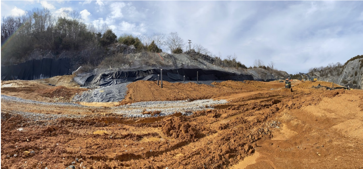
Figure 1. Phase 1 Sidewall Odor Mitigation System Construction
