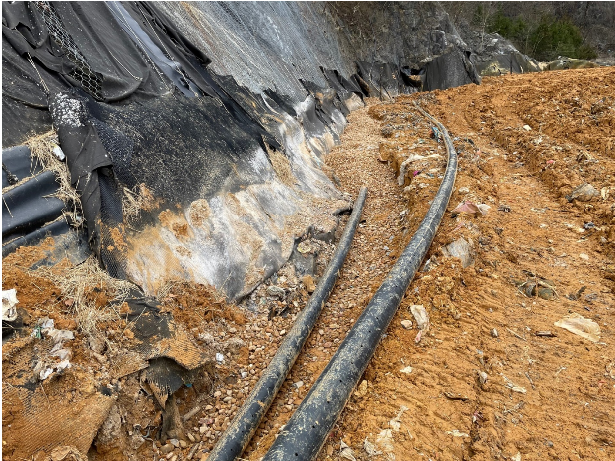
Figure 2. Phase 2 Sidewall Odor Mitigation System Construction
