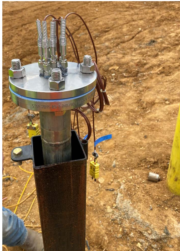
Figure 3. In-waste Temperature Sensor Installation
