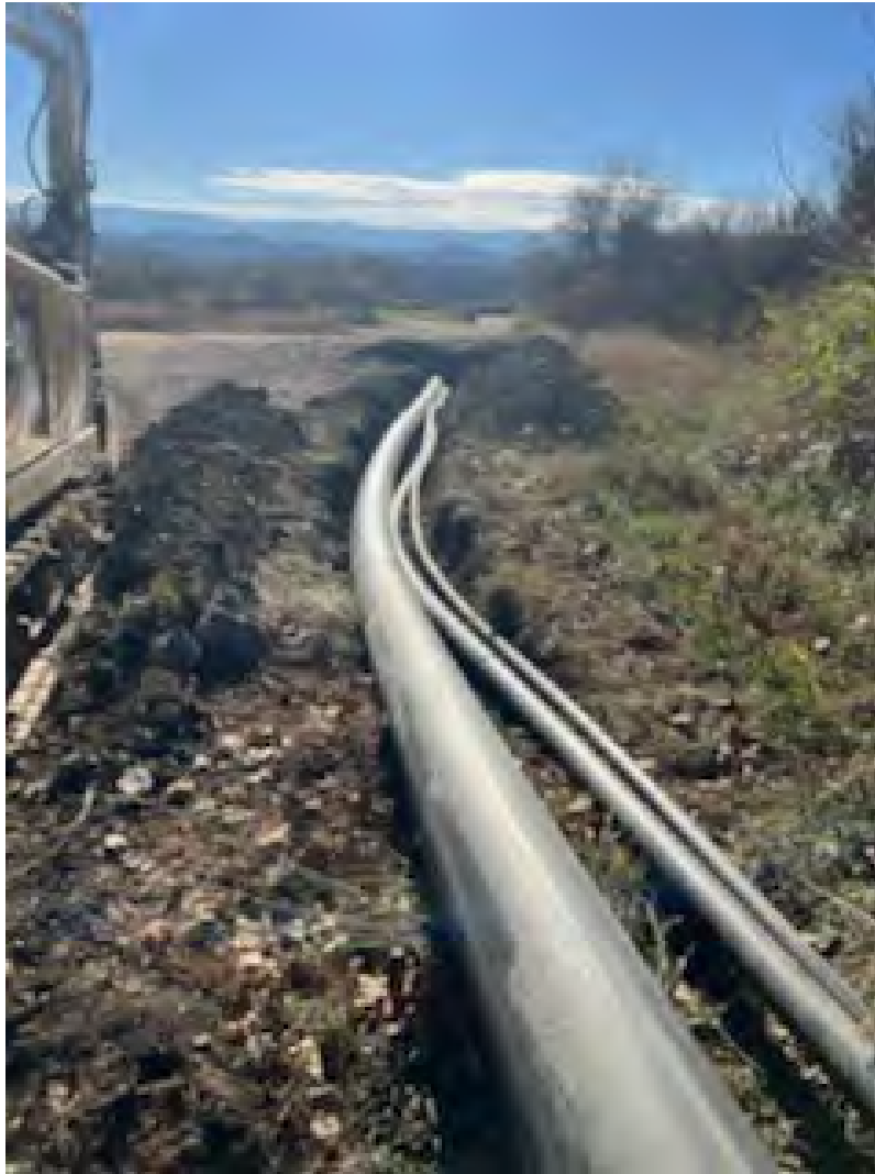
Figure 2. Installation of 12-inch Header, 2-Inch Airline, and 4-Inch Forcemain in Common Trench
