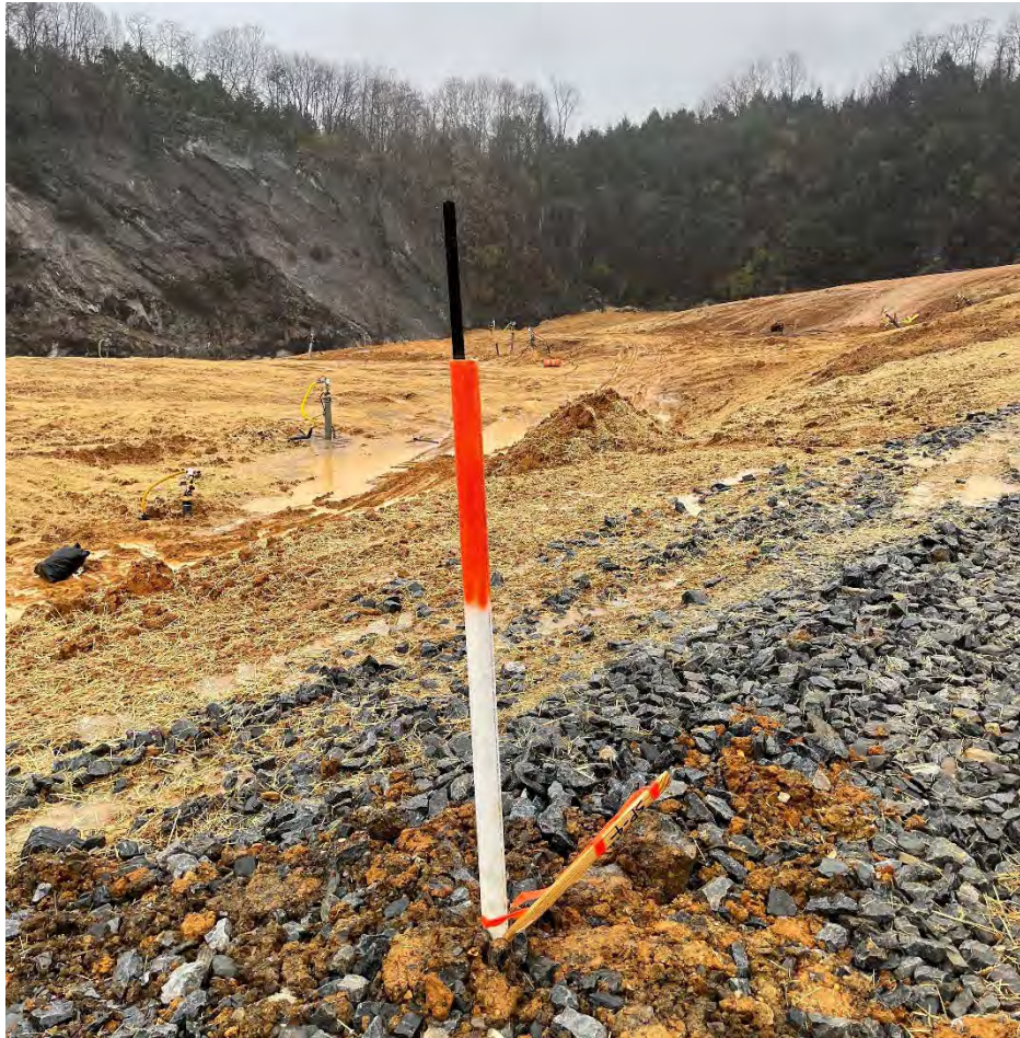
Figure 12. Settlement Plate after Installation
