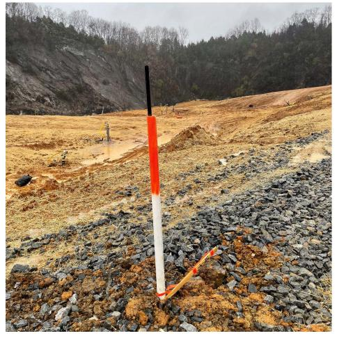
Figure 3. Settlement Plate after Installation
